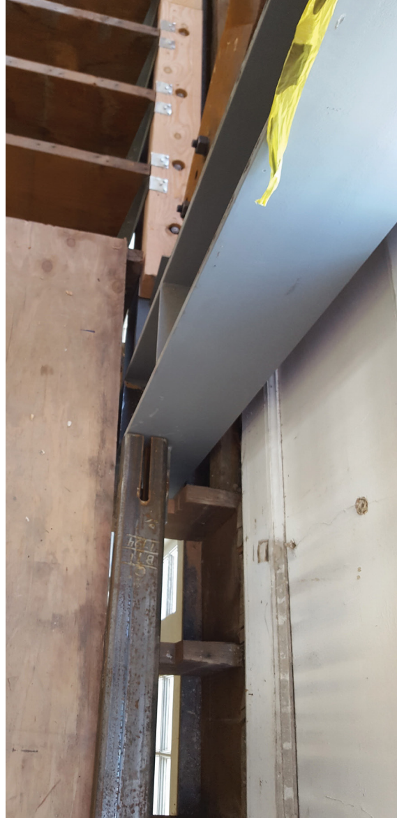
HSS collector recessed into the top of floor framing.
