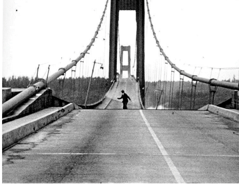
Photographer Howard Clifford, escapes the Tacoma Narrows Bridge during collapse.
