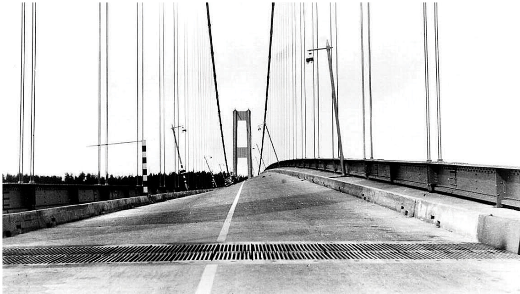
Tacoma Narrows Bridge twisting prior to collapse.
