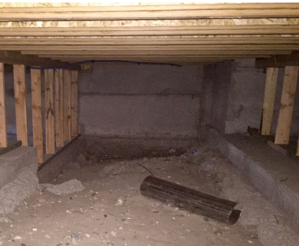
Figure 5. Interior cripple walls.
